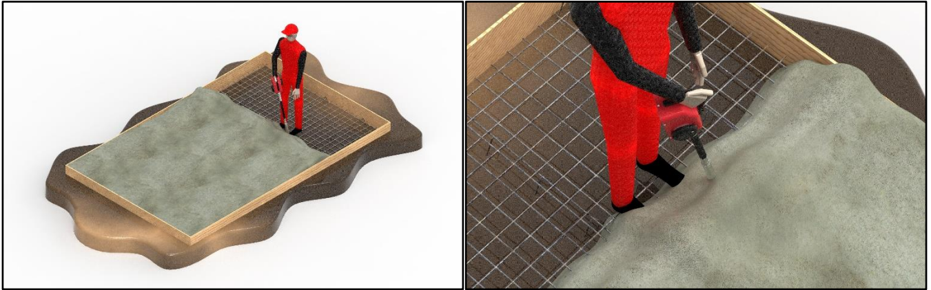
Figure 6: Operation procedure during the compacting of concrete.
